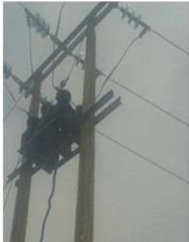
Plate 6.1 pole mounted boundary Meter [26]
