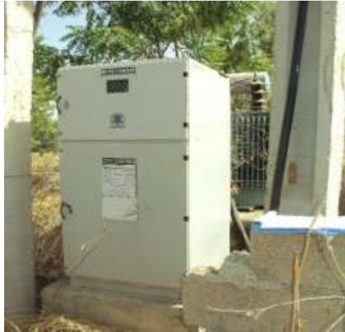
Plate 6.2: Distribution Transformer Metering [26]
